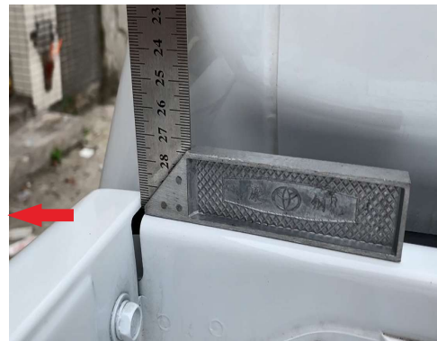
Check if the side bars and the front middle bar are horizontal before installing
